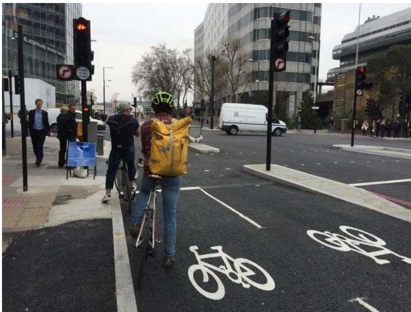
Fig. 22: Kerb separated two-way cycle track with its own signals. Blackfriars Road, London.
