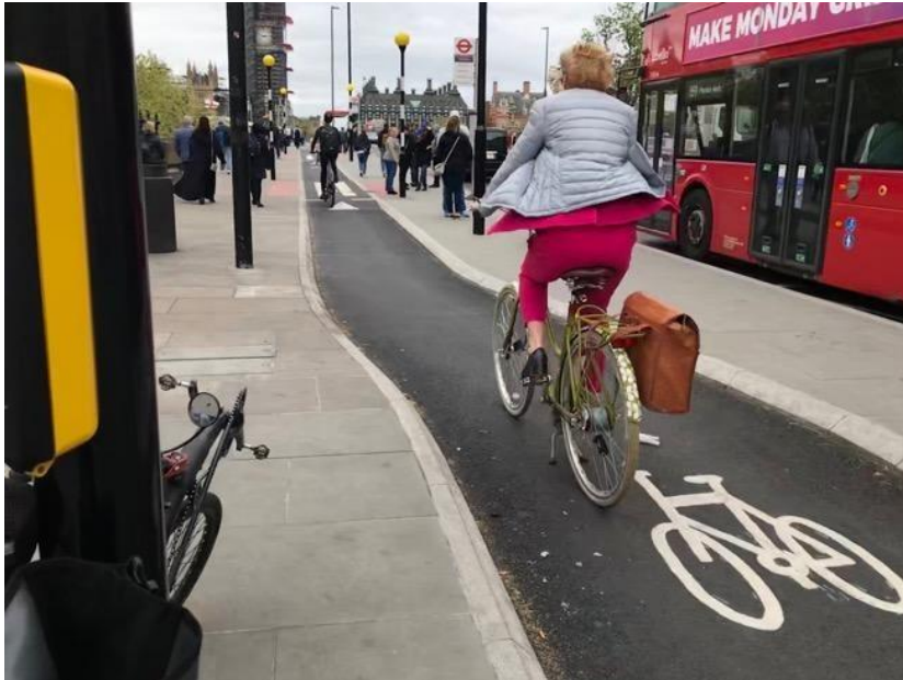
Fig 24: Bus stop bypass. Efforts should be made to minimise conflict between cycles and pedestrians.
