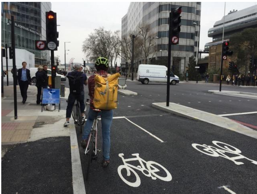
Fig. 22: Kerb separated two-way cycle track with its own signals. Blackfriars Road, London.
