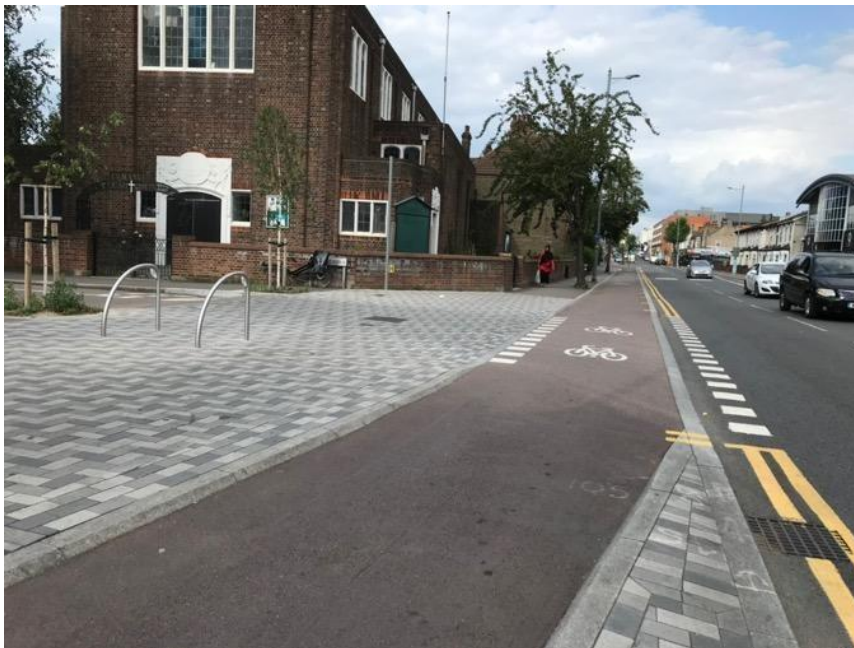
Fig 23: A cycleway crossing a side road junction alongside a continuous footway. Drivers must give way to pedestrians and cyclists using this junction (Highway Code).
