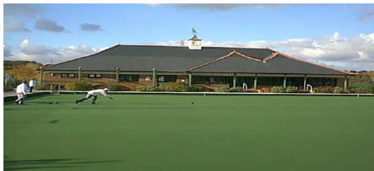
A Totton & Eling Town Council Facility
